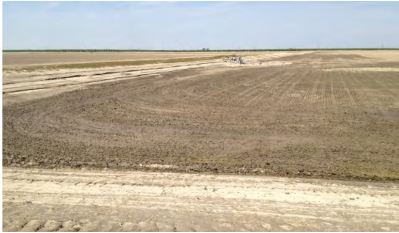
View of existing Stockdale West recharge basin
