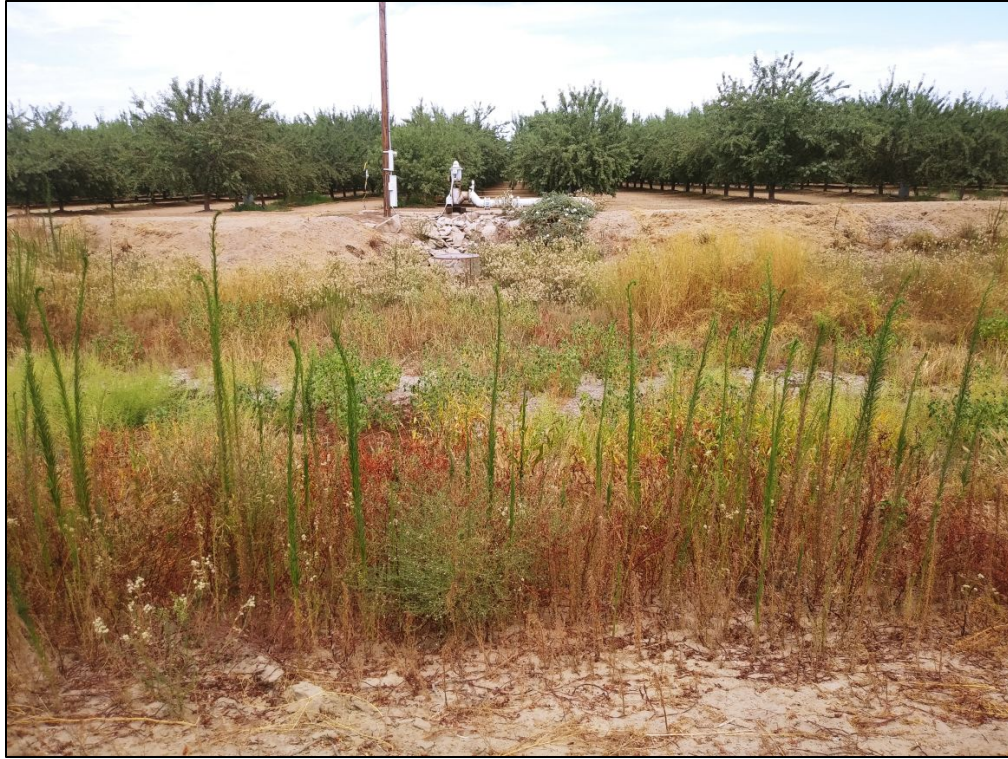
Figure 4b. McCaslin weir and intake area, looking north.
