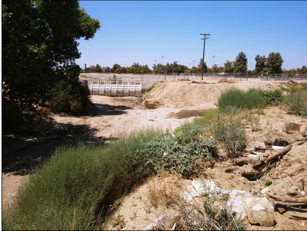
Figure 4d. Kern River and Cross Valley Canal intake improvements area, looking west.
