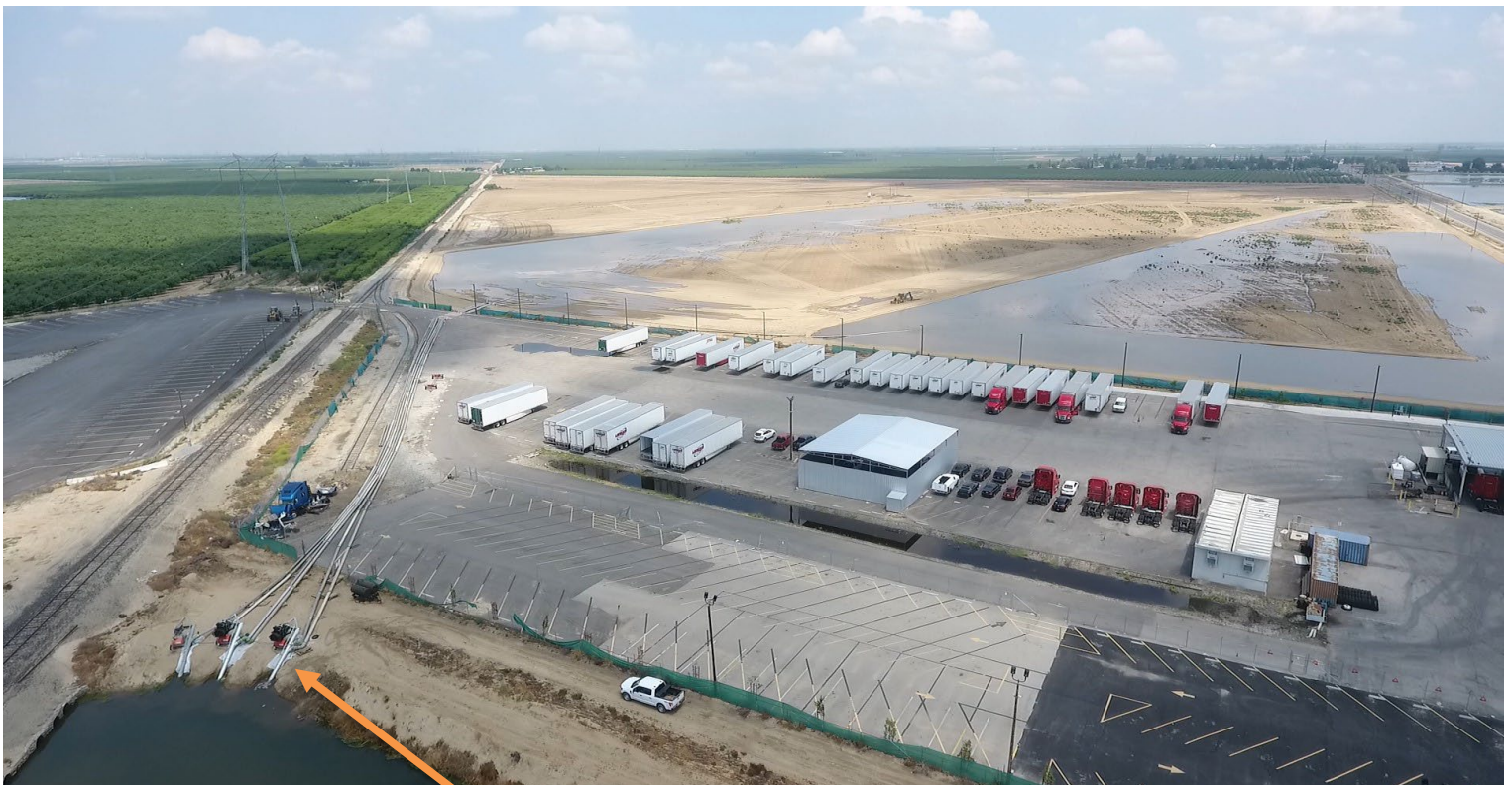
(3) 16" Pumps on Goose Lake Channel. Estimate = 40 cfs
