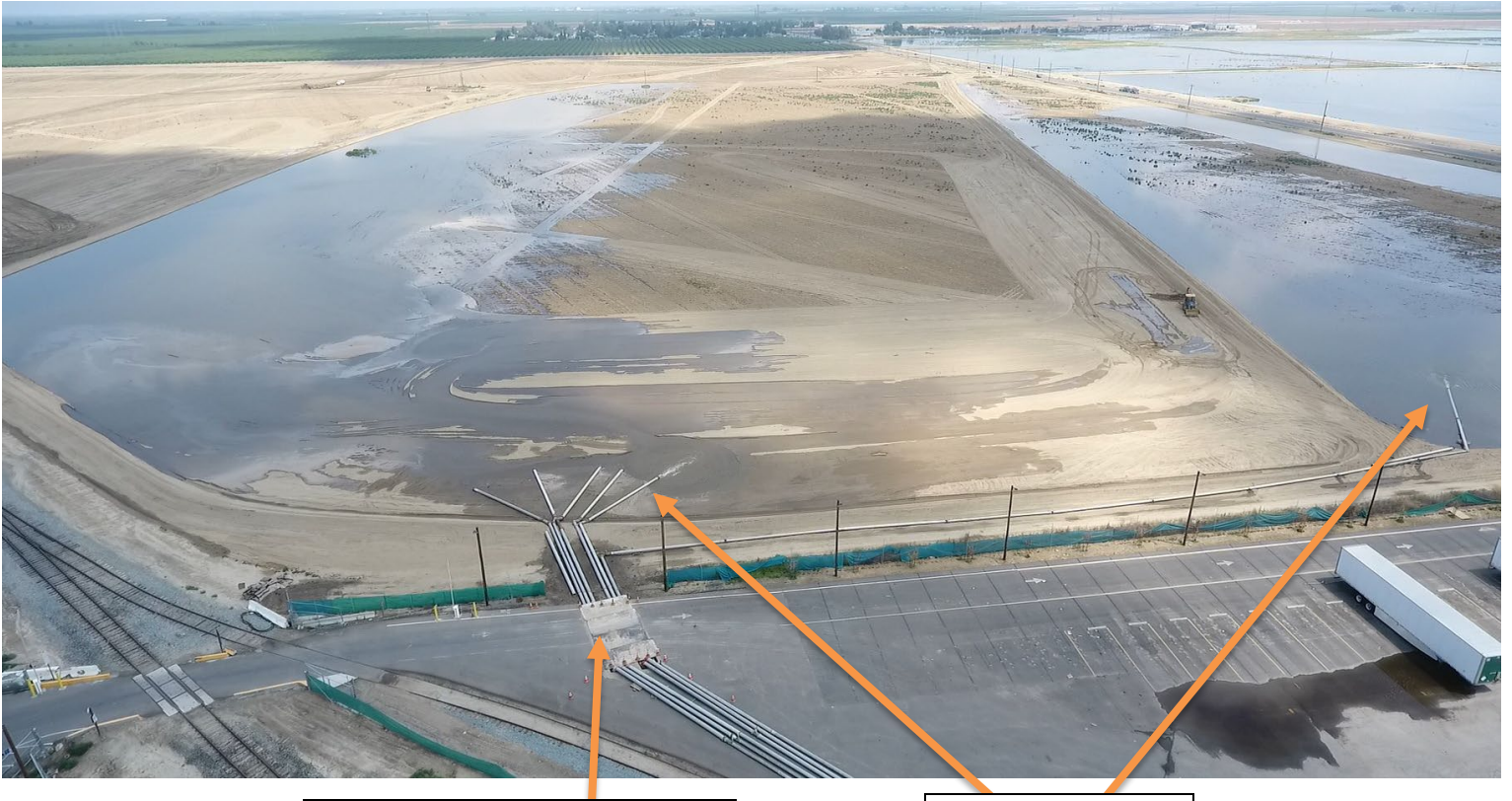
Steel Plates allowing for truck access to back lot.
