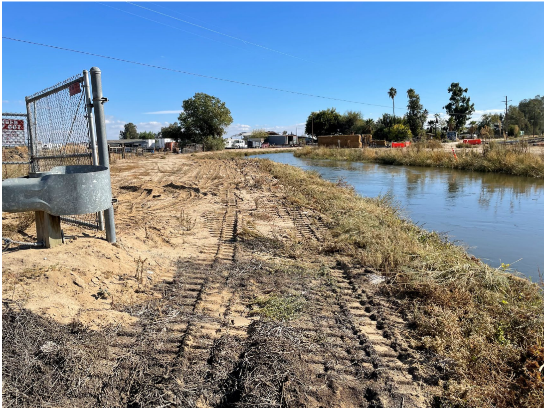
Channel south of Brimhall Road – Before & After
