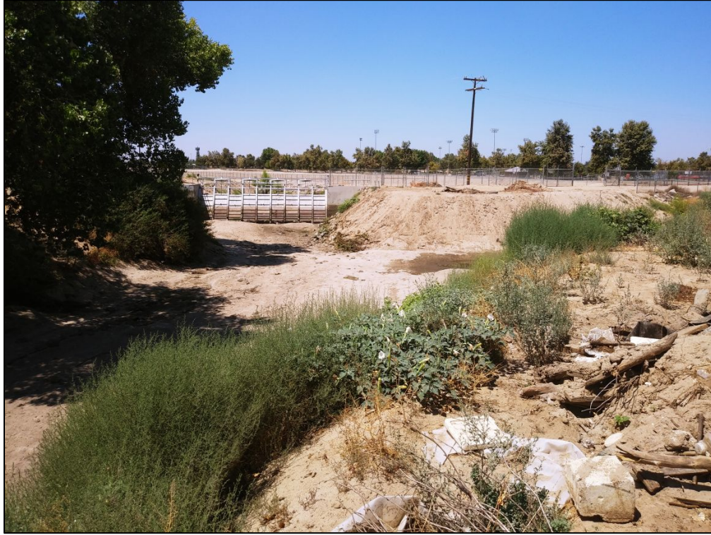
Figure 4d. Kern River and Cross Valley Canal intake improvements area, looking west.
