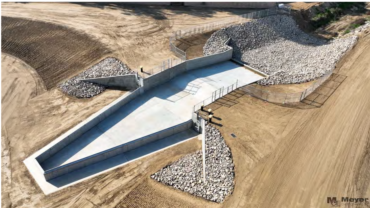
Houghton Weir Reconstruction Project
