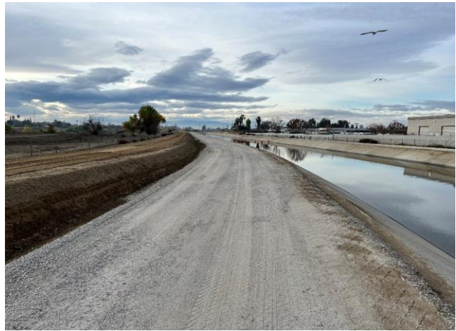
Ag base road placed.
