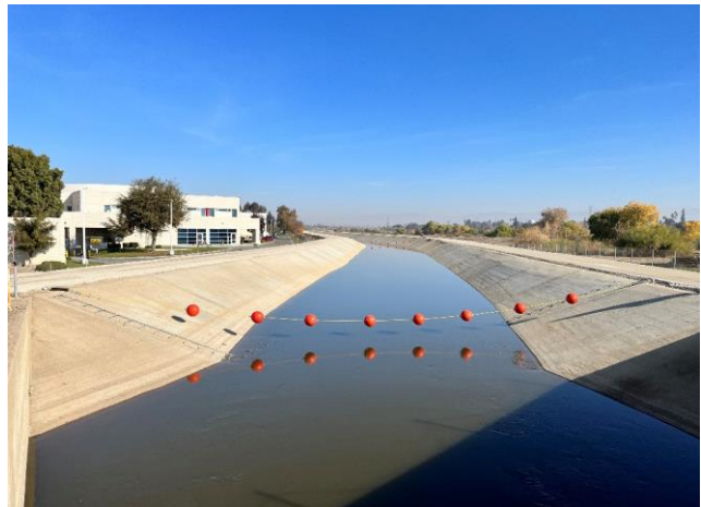
View north of siphon.
