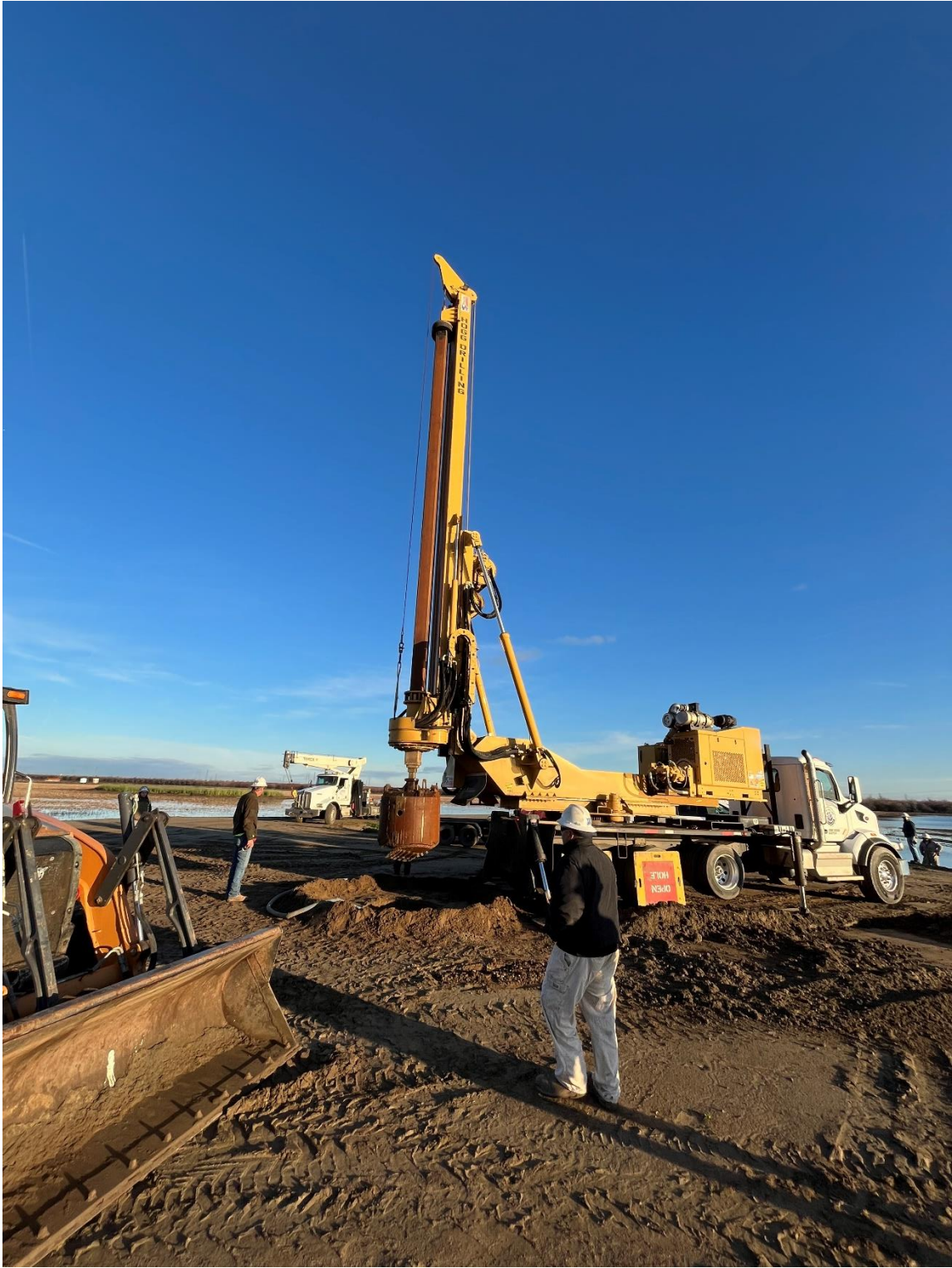
Figure 1: Drilling of initial conductor hole approx. 40" diameter
