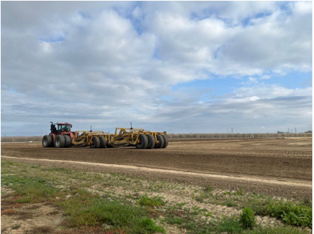
Placement of Fill on Westerly Levee of Basin 3
