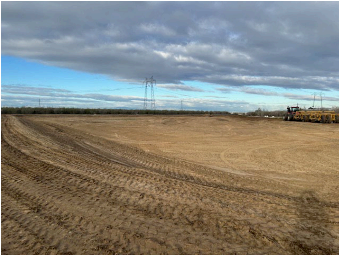
Filling and Compaction of Basin 4 Levee Embankment
