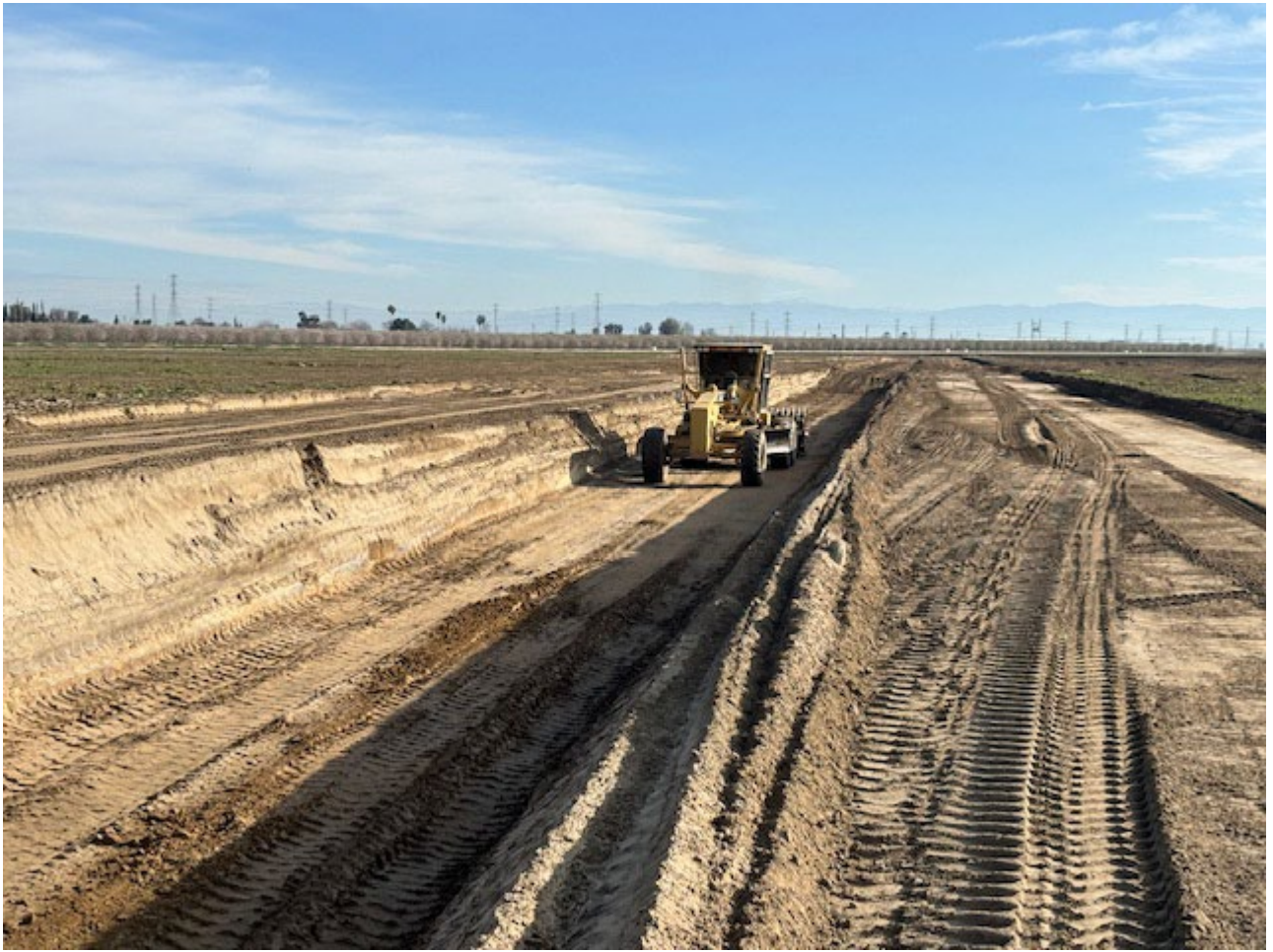
Scarifying and Compacting Keyway in Southeasterly Levee of Basin 3
