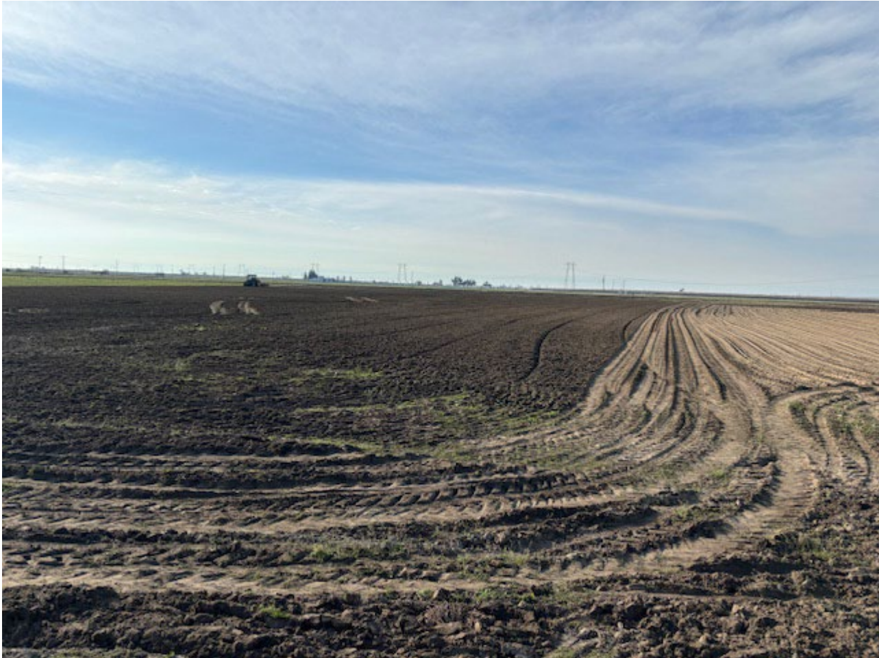
Clearing and Grubbing in Basin 2
