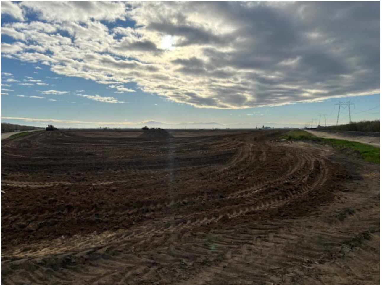
Filling and Compaction of Levee in Northwest Corner of Basin 4
