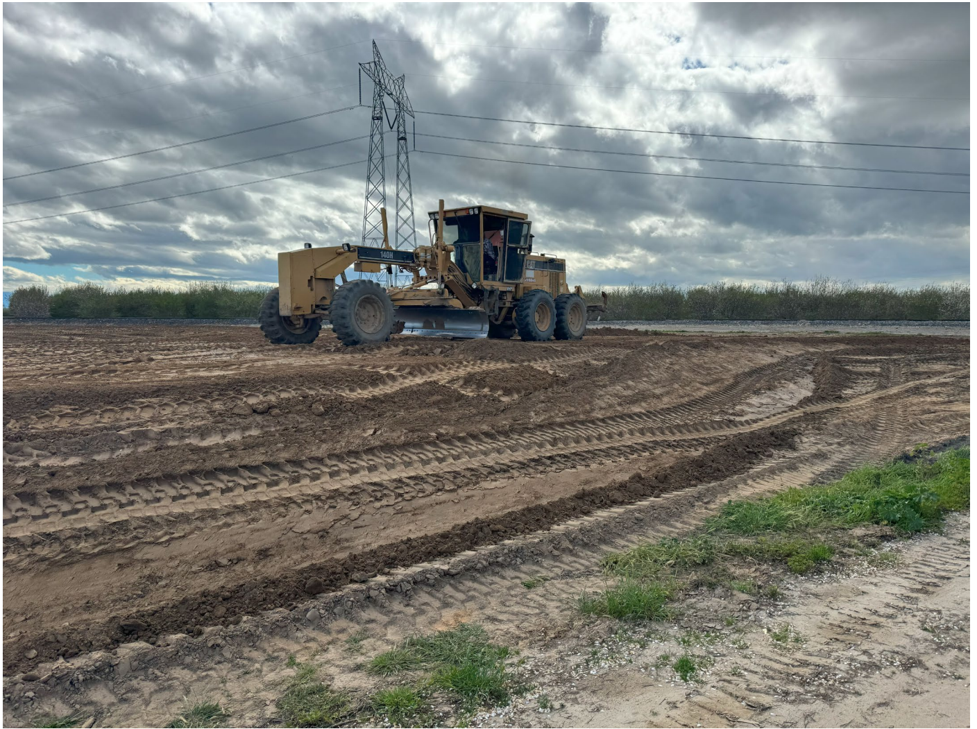
Fine Grading the Slopes and Top of Embankments at Basin 4
