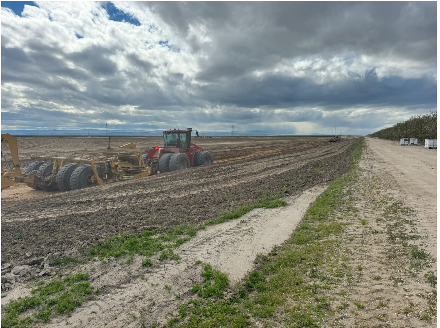
Excavating Keyway for North Levee of Basin 2
