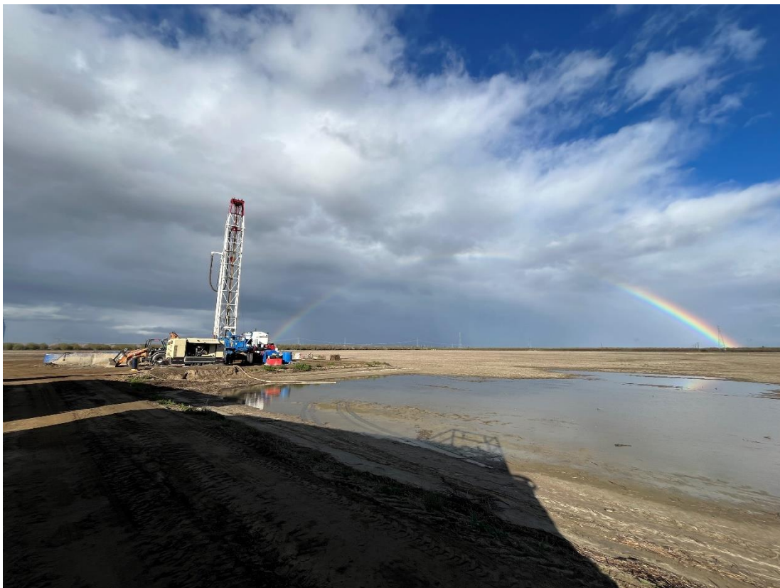
Figure 4: Example of zone sampling. Certain depths are sealed off, pumped on, and tested for water quality
