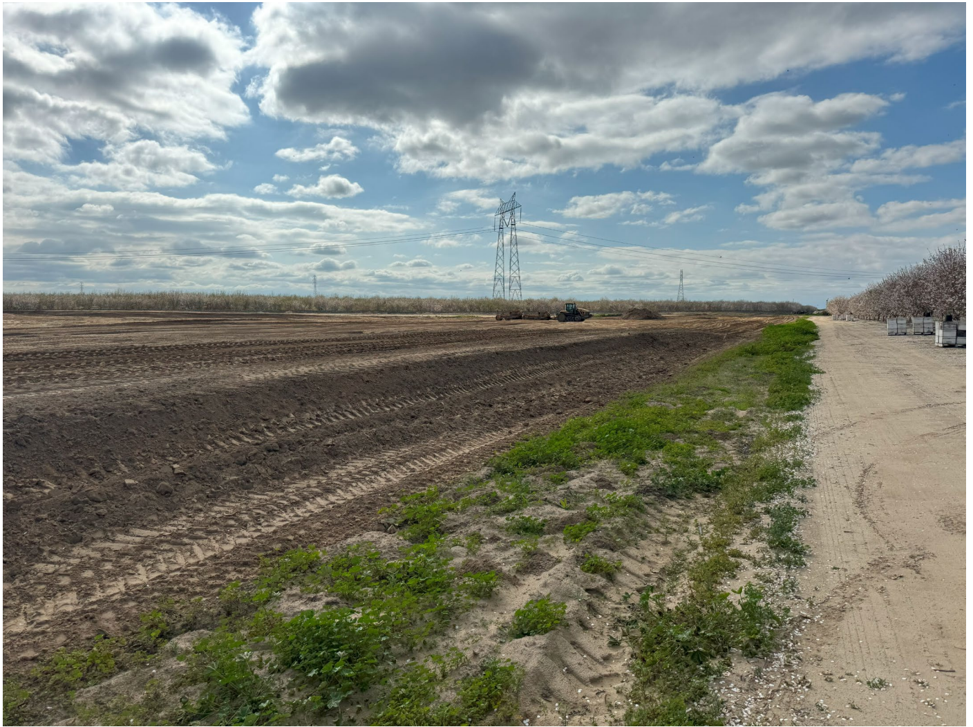
North Levee for Basin 4
