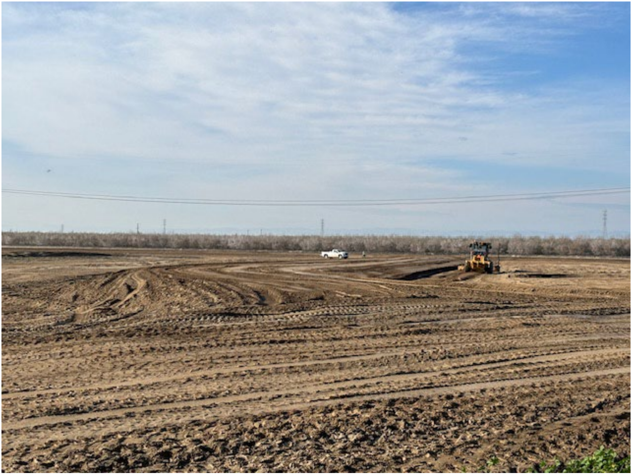
Filling and Fine Grading Levee Embankment in Basin 4
