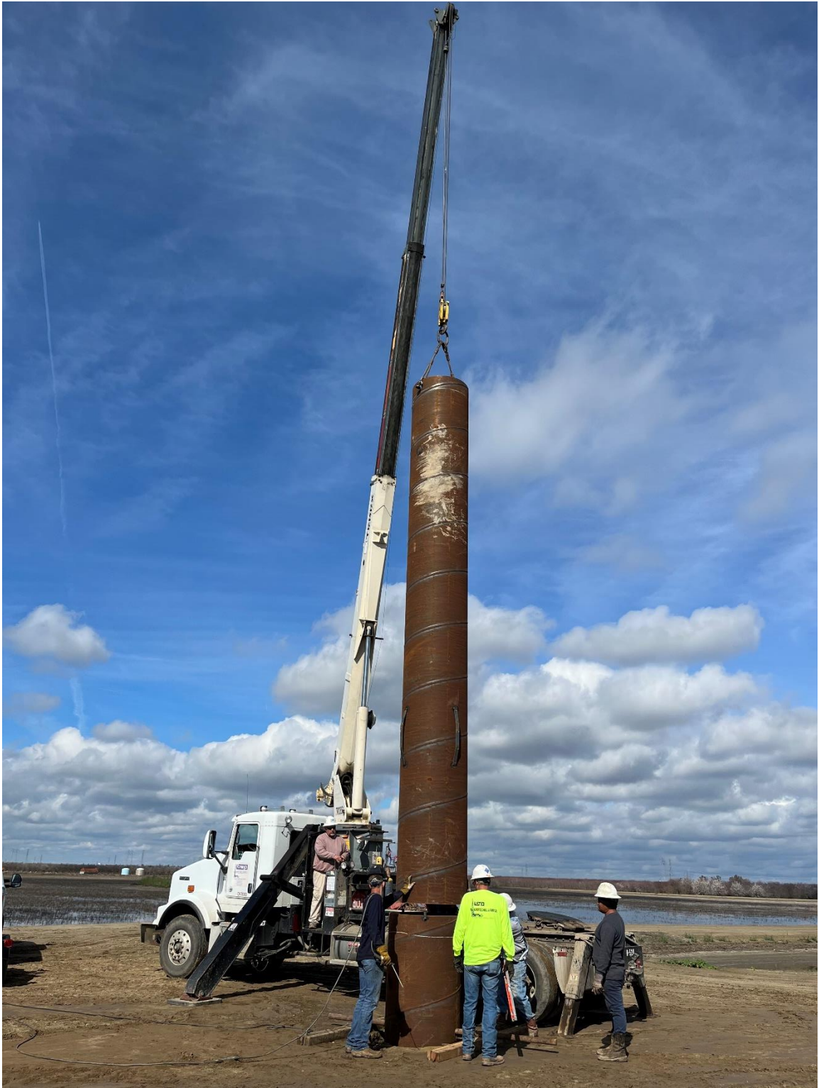
Figure 2: Setting of conductor (36") at McCaslin 2
