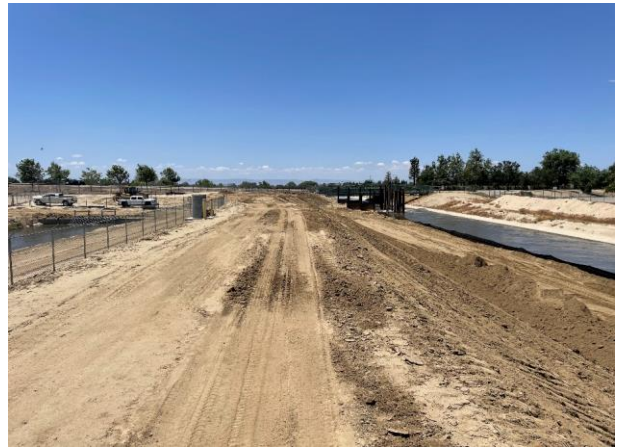
Plates within canal prism removed and slope armored with rip-rap.
