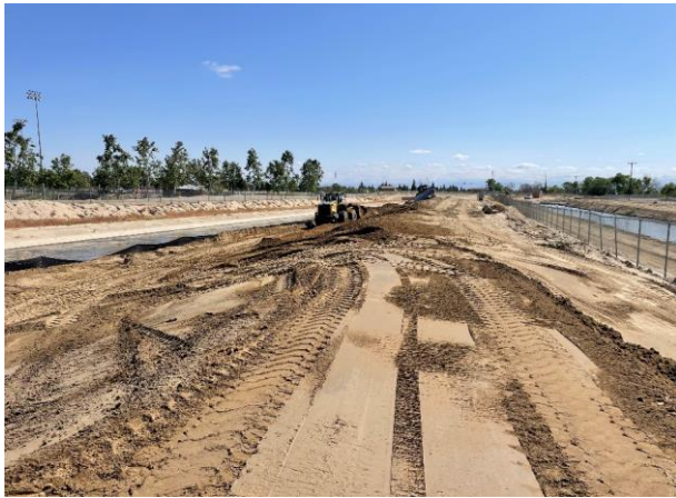
Removing plates from shoring system.
