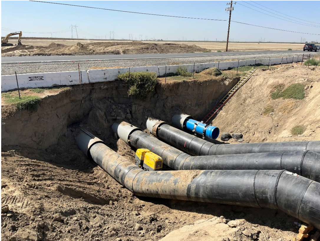
Installation of 42" HDPE Pipe Underneath Enos Lane (State Route 43)
