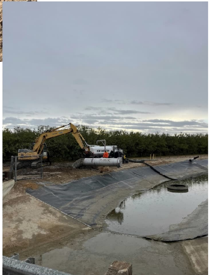
Installation of McCaslin/Bowling Recovery Pipeline
