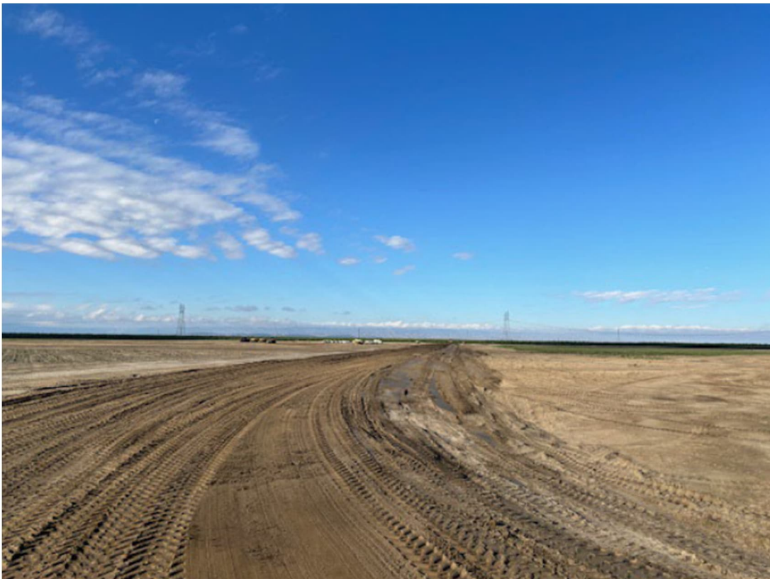
Construction of Levee Embankments
