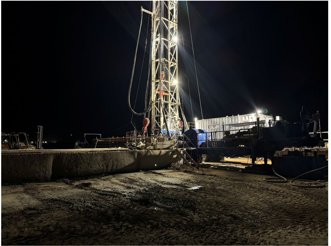
Rig During Airlifting and Swabbing Process
