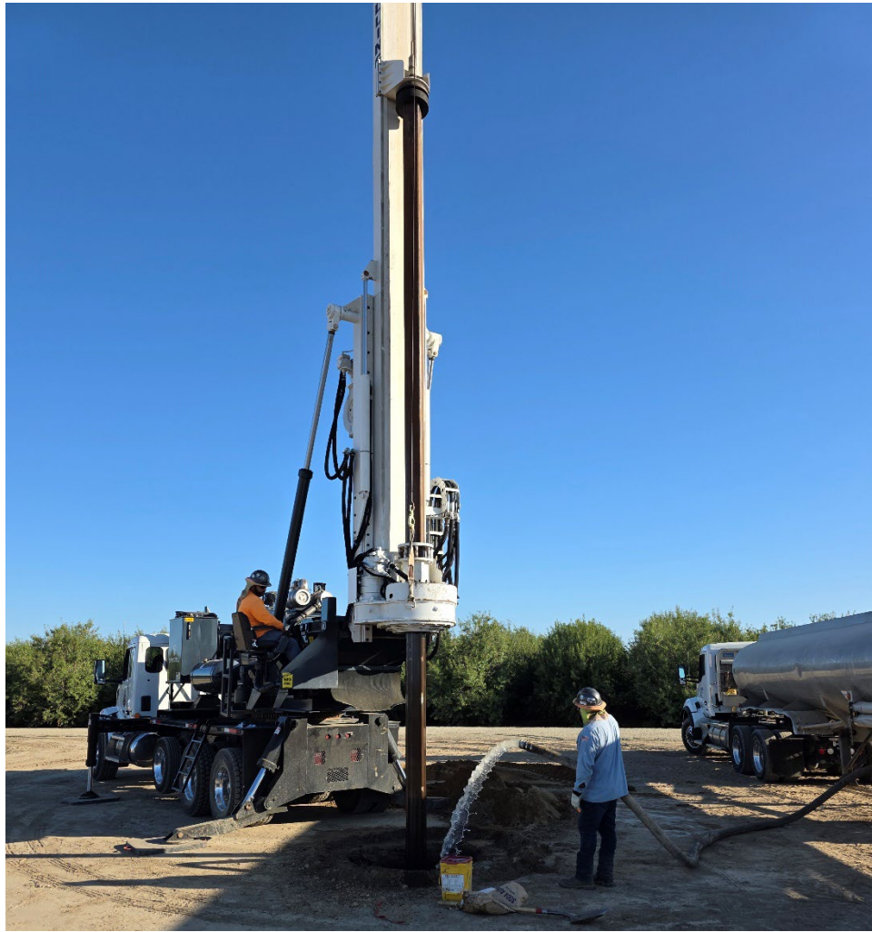
Conductor Casing Drilling
