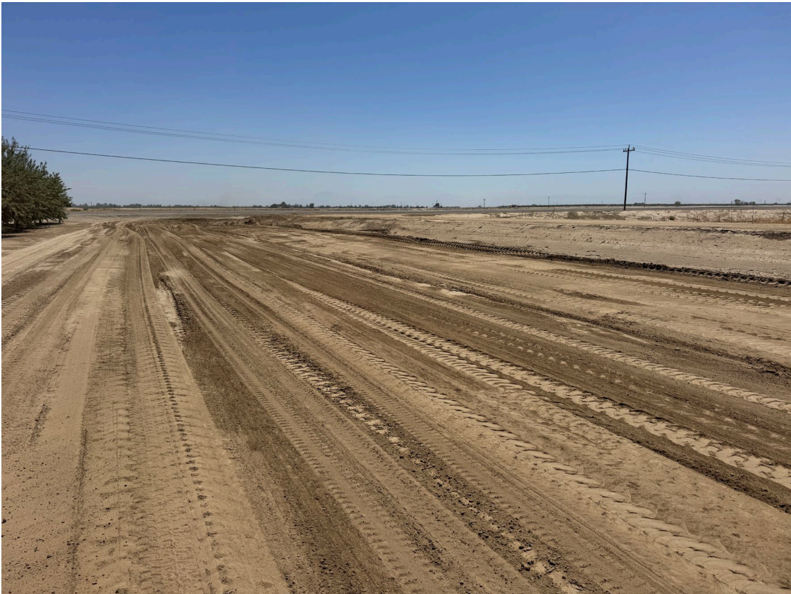
Fine Grading of Pipeline Alignment
