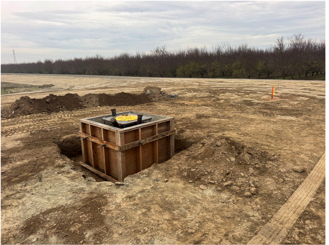
Well Foundation at SN-1
