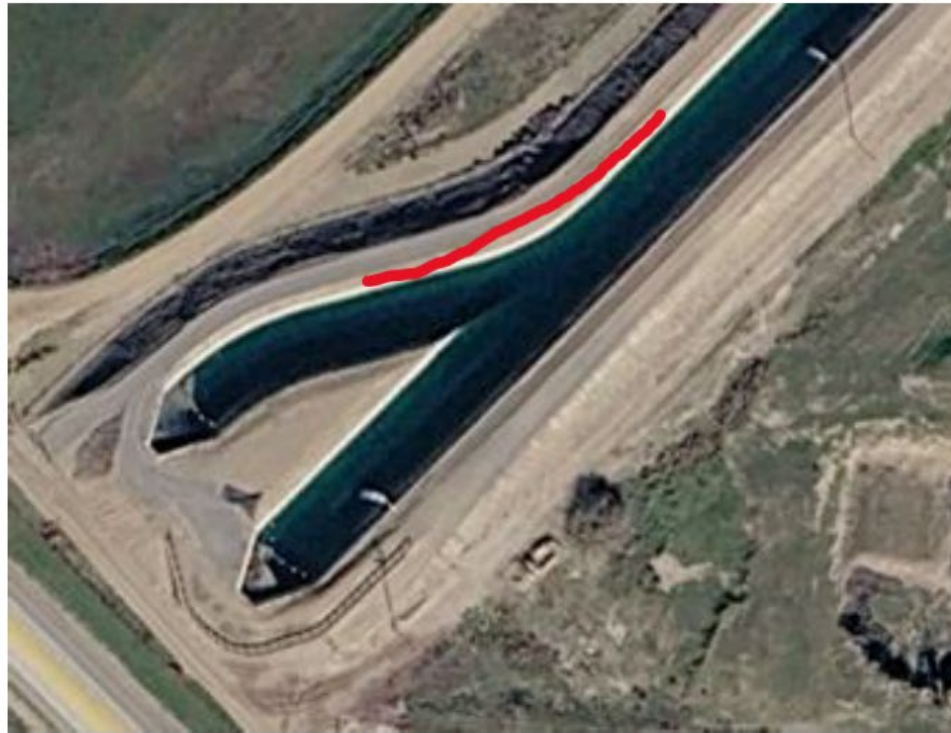
Figure 3. PP1 afterbay after I5 siphon needs to have a wider smoother transition to the main pool.
