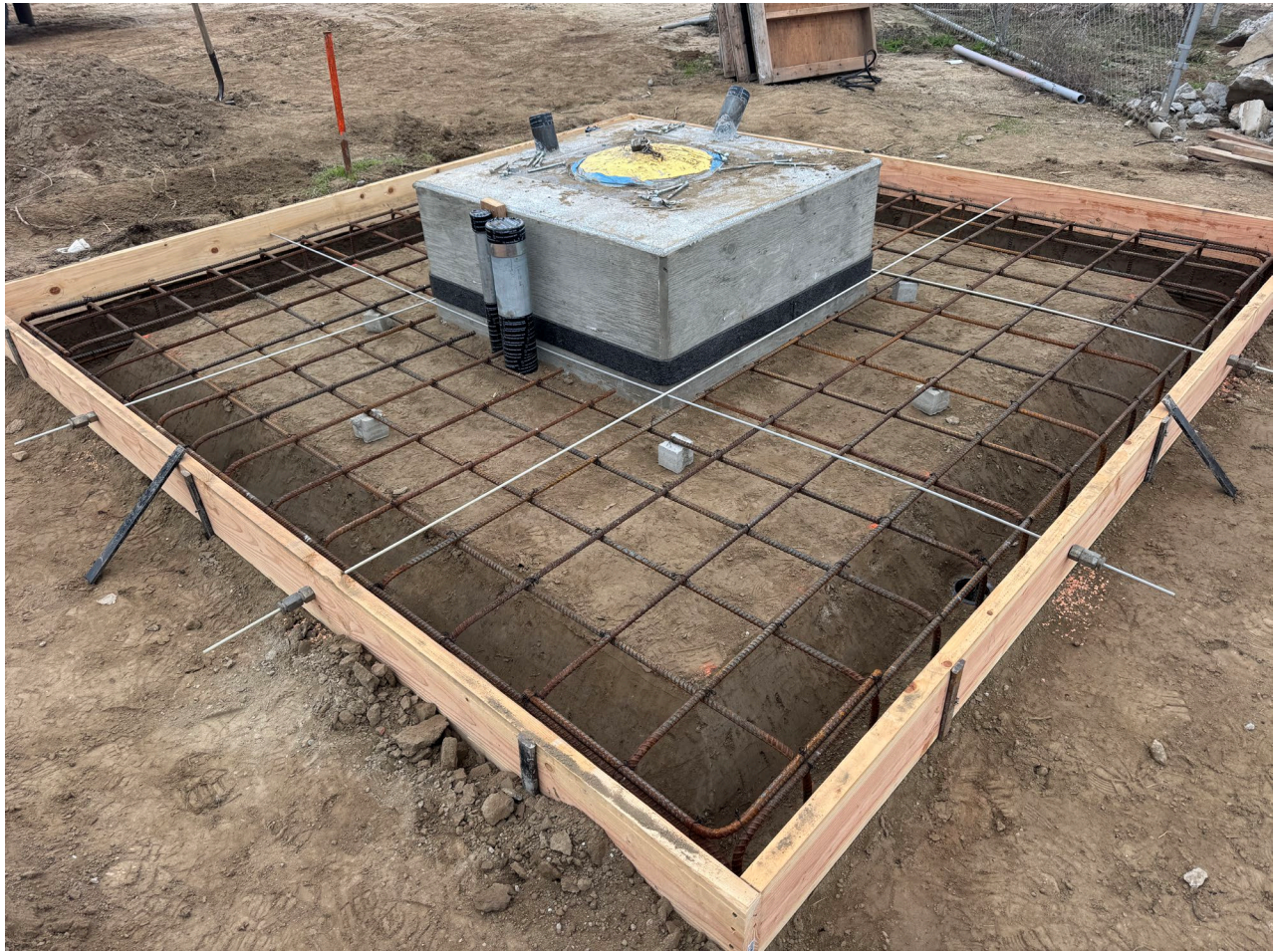
Well Foundation at WE-AG
