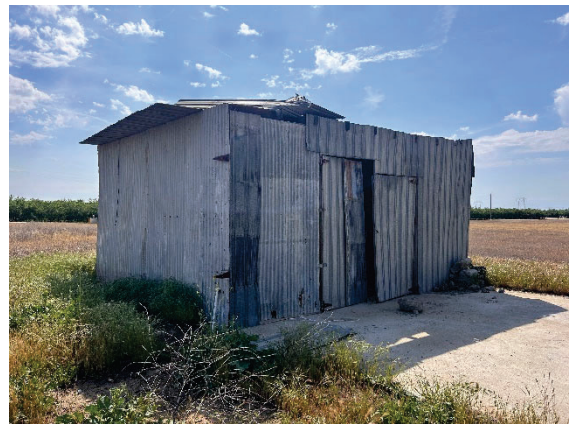
Photo #6 View of the structure on Site, facing southeast.
