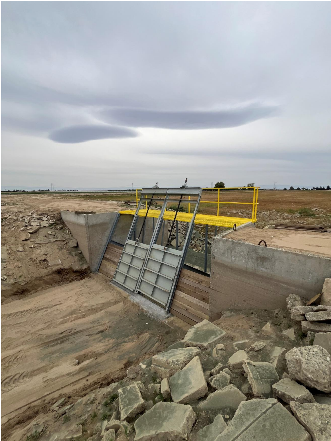
Figure 5 West Superior Weir Complete
