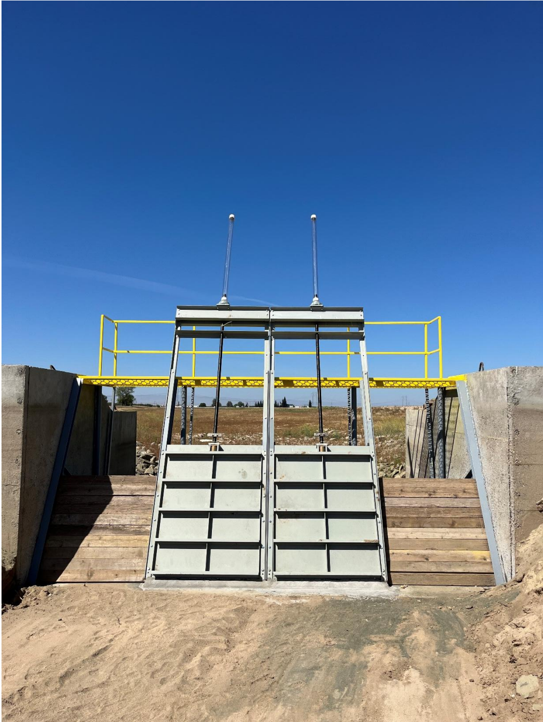
Figure 4 West Superior Weir front view
