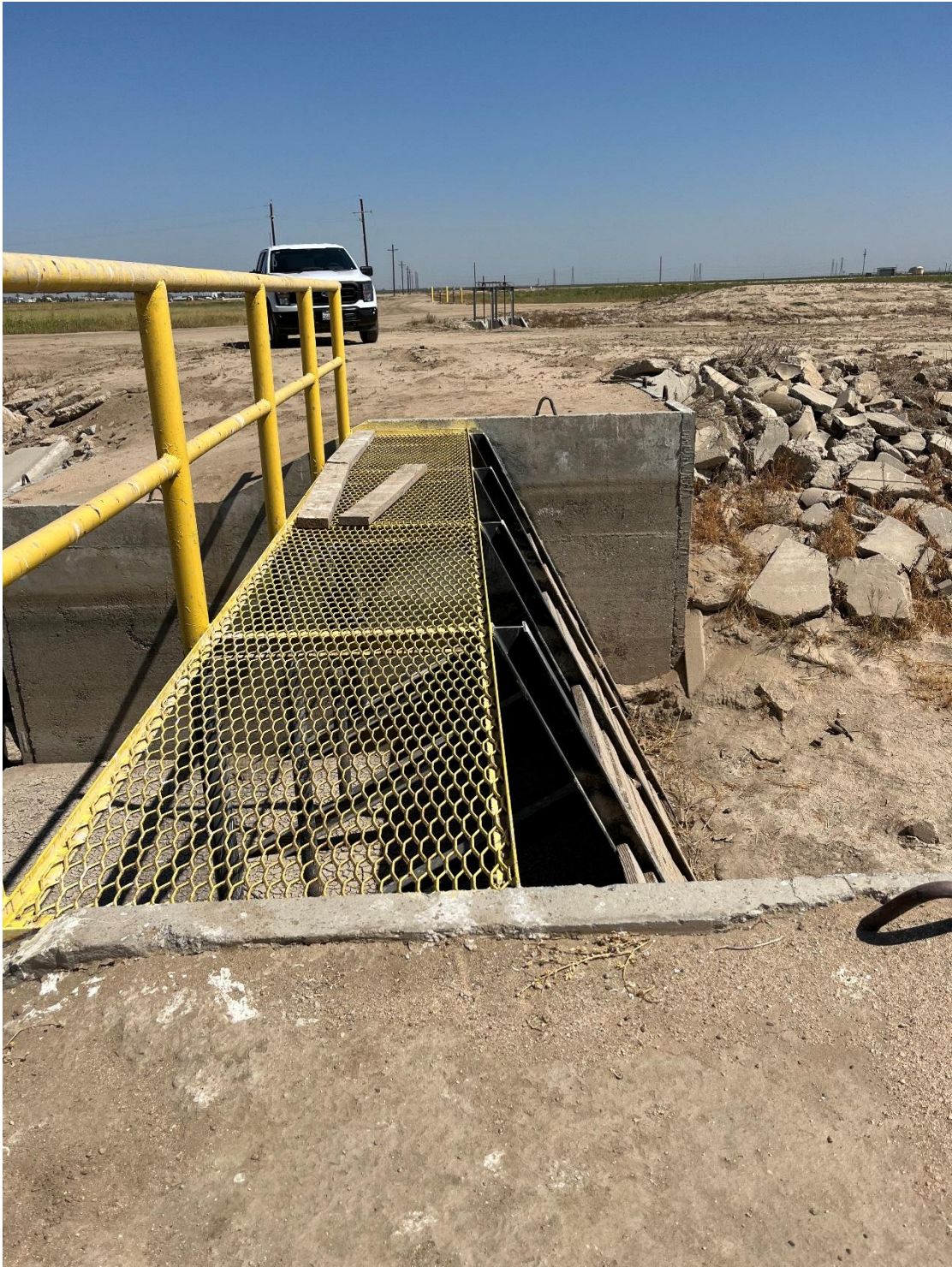
Figure 2 West Superior Weir before modifications
