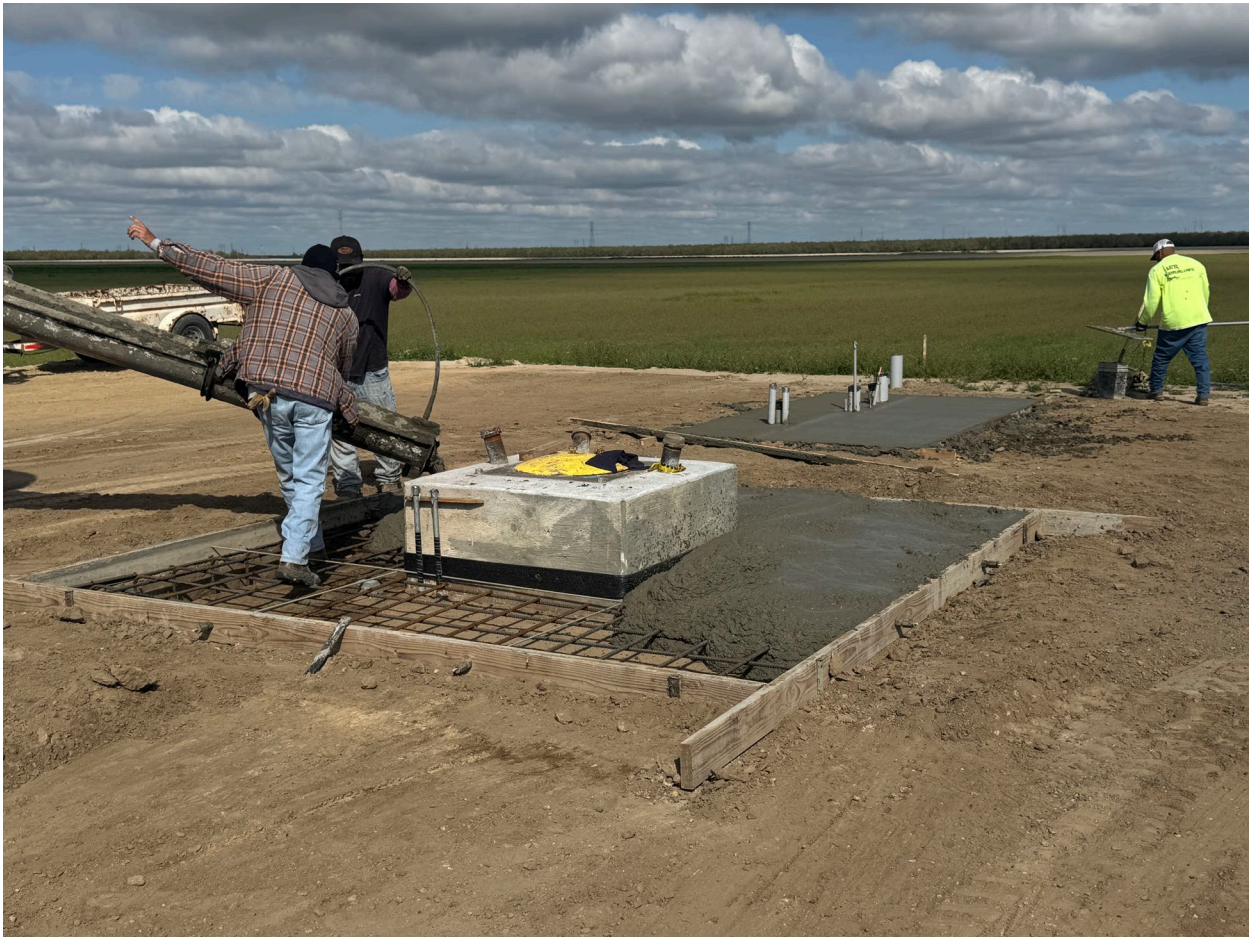
Placement of Concrete around Well Foundation at SN-2
