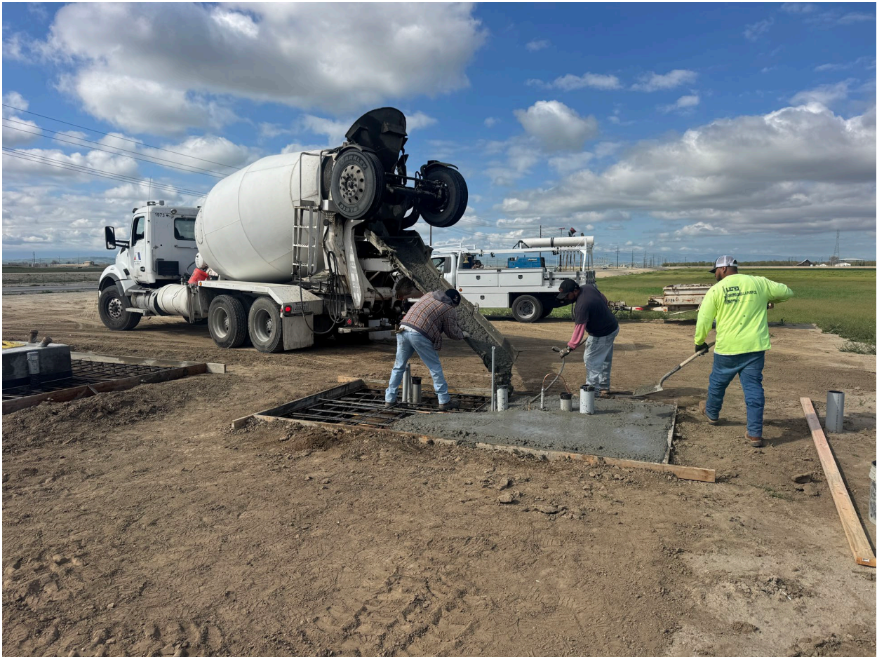
Placement of Concrete for Electrical Pad at SN-2
