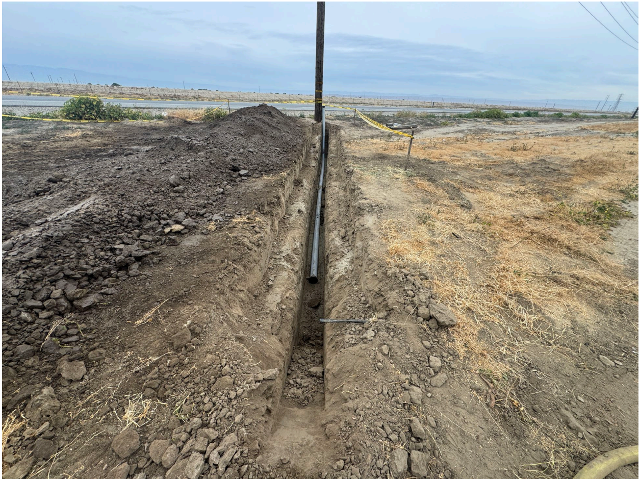
Conduit Installation for Electrical Service at SN-2
