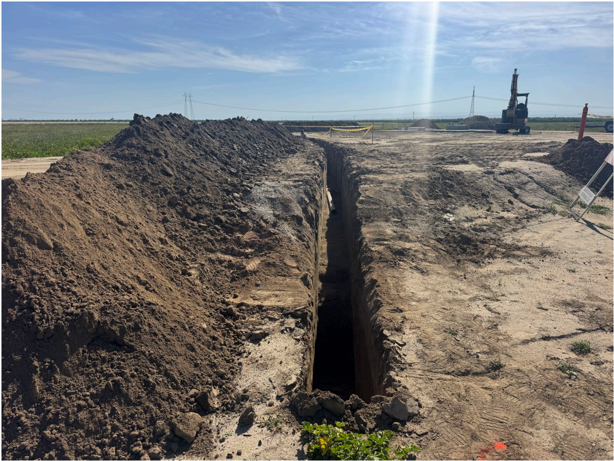
Trench Excavation for Electrical Service
